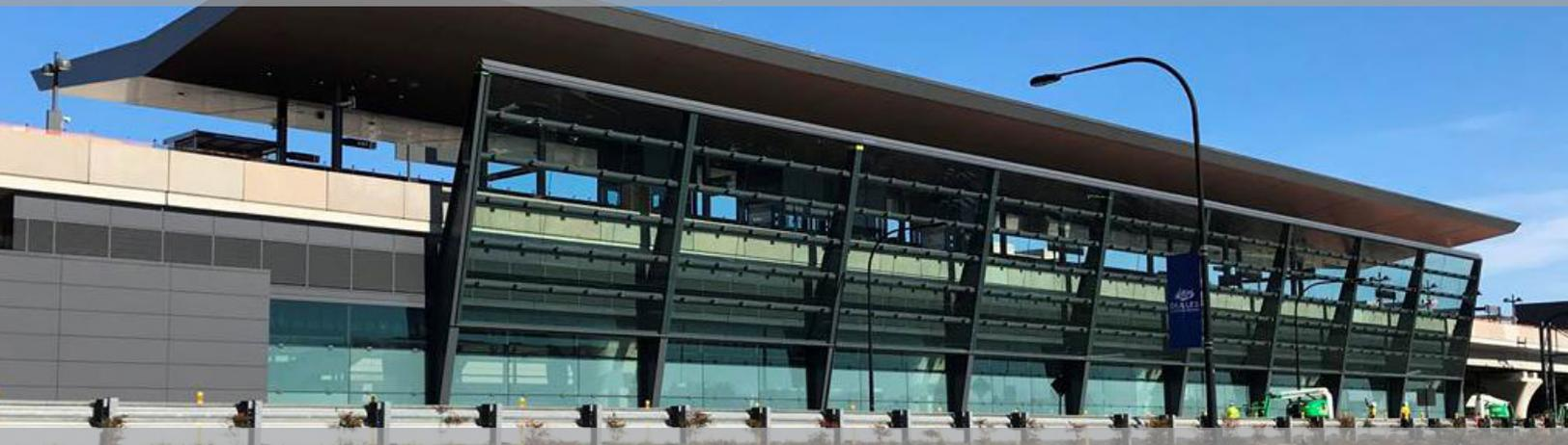
Crews with W.M. Schlosser have finished installing glass panels that will comprise the windscreen at Dulles Airport Station that was designed to mimic the facade Dulles International Airport. (Photo courtesy of Dulles Corridor Metrorail Project)
