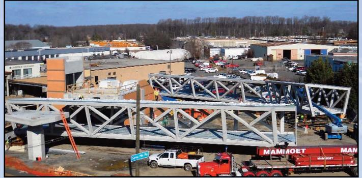
READY FOR LAUNCH: Spans for the pedestrian bridges at the Spring Hill (Tysons West) Station were assembled in preparation for erection across eastbound and westbound lanes of Route 7. *Photo by Stephen Barna, Dulles Corridor Metrorail Project*
