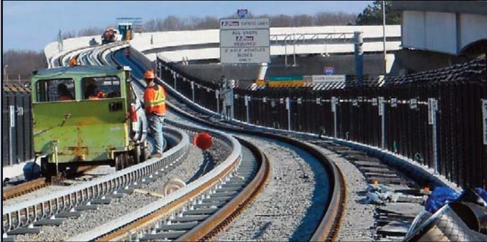
ON THE TYSONS WEST GUIDEWAY LOOKING NORTHEAST: Construction of walls, track bed, track and security fences are complete. *Photo by Stephen Barna, Dulles Corridor Metrorail Project*
