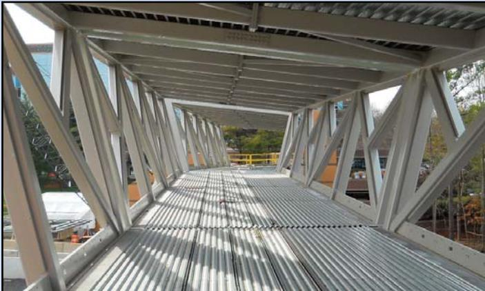
INSIDE A PEDESTRIAN BRIDGE AT WIEHLE STATION: Pedestrian bridge spans have been erected and await interior and exterior finishing. *Photo by Stephen Barna, Dulles Corridor Metrorail Project*
