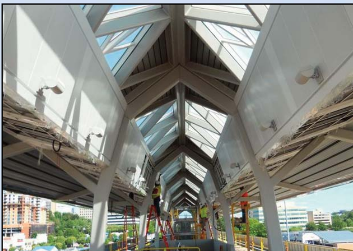
SILVER LINE WORK CONTINUES IN TYSONS: Finishing work continues at the Spring Hill Metrorail Station. Here the roofing system skylights, ceiling panels and light on the platform canopy are being installed. Platform pavers are complete. Platform light and windscreen installation will begin soon. This photo is looking east along Route 7. Photo by Stephen Barna, Dulles Corridor Metrorail Project
