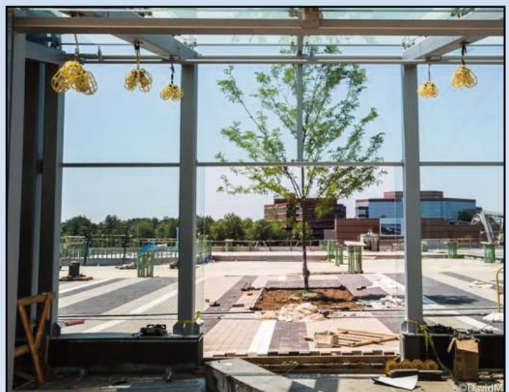
SILVER LINE WORK CONTINUES IN TYSONS: Finishing work continues at the Spring Hill Metrorail Station. Here the roofing system skylights, ceiling panels and light on the platform canopy are being installed. Platform pavers are complete. Platform light and windscreen installation will begin soon. This photo is looking east along Route 7. Photo by Stephen Barna, Dulles Corridor Metrorail Project
