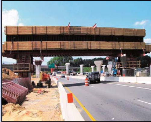
The straddle bent over westbound I-66 just after the Dulles Connector Road interchange. Photo by Dulles Corridor Metrorail Project
