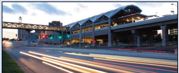
DAZZLING LIGHTS ON ROUTE 123: Car lights, traffic signals and lights within the pedestrian bridge at the Tysons Corner Station illuminate this busy road. Photo by Chuck Samuelson, Dulles Corridor Metrorail Project
