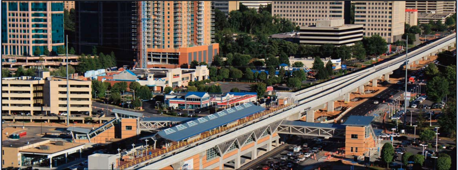
DIFFERENT LOOK: Dulles Rail Project photographer Chuck Samuelson captured the changing landscape of Route 7 near the Spring Hill Station from atop the Sheraton Hotel.
