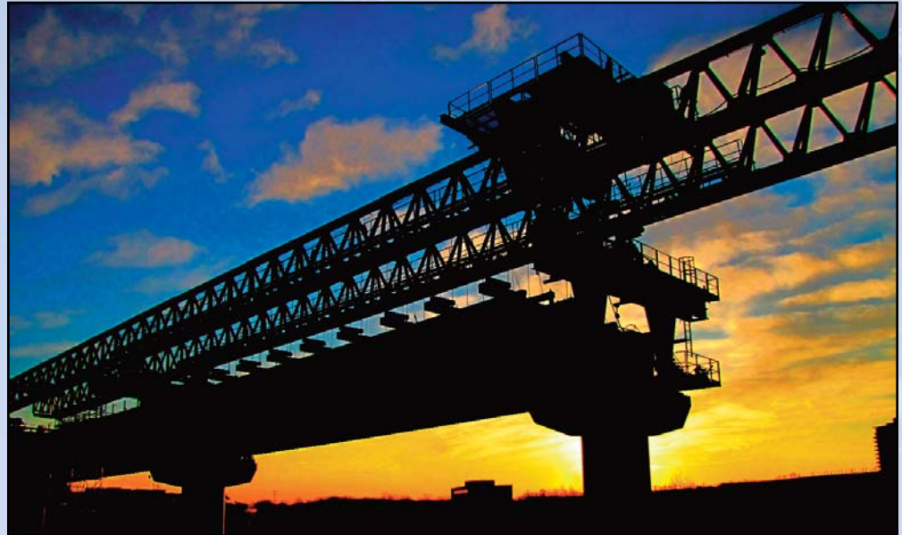
AS MORNING LIGHT BREAKS: One of three horizontal cranes is silhouetted against the morning winter skies along Route 123 in Tysons Corner. Photo by Chuck Samuelson, Dulles Corridor Metrorail Project
