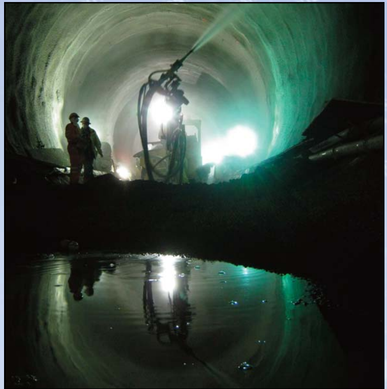
REFLECTIONS: Crews spray concrete on to the surface of the tunnels. Mining on both the inbound and outbound tunnels are complete, and the next phase of tunneling work is expected to last one more year. Photo by Frank Jenkins, Dulles Transit Partners
