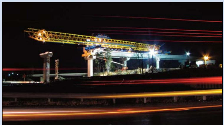
LIGHTING UP THE NIGHT SKIES: Crews build bridge spans using a horizontal crane near Route 123. Below the structure, traffic along Interstate 495 generates brilliant streams of color. Photo by Chuck Samuelson, Dulles Corridor Metrorail Project
