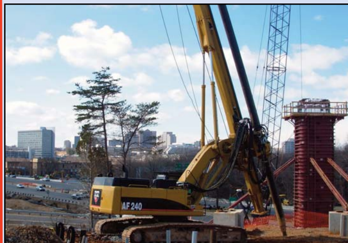
Pier construction at the Dulles Connector Road and Route 123 interchange leading up to the future Tysons East Station. Photo by Dulles Corridor Metrorail Project
