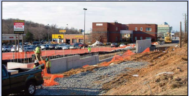
Construction of retaining walls on Route 7, necessary to build up the service roads to the same grade as Route 7 for lane shifting. Photo by Dulles Corridor Metrorail Project
