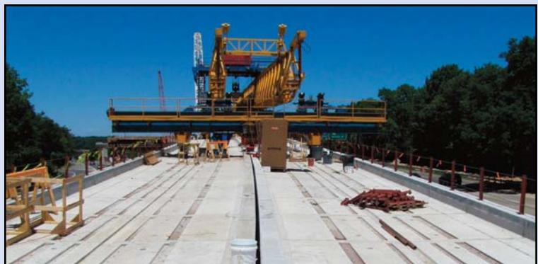
The first truss, located in the median of the Dulles Connector Road (Route 267) near the Route 123 intersection, continues guideway construction as it moves closer to Route 123. Photo by Dulles Corridor Metrorail Project
