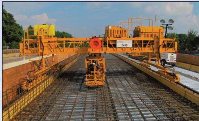
Civil crews have been working on several bridges over roads, trails and streams. This bridge work over Magarity Road in the median of the Dulles Connector Road (Route 267) is the beginning of some of the superstructure work, which requires massive amounts of rebar, concrete and system support. These bridges are part of the at-grade portions of the track that will eventually carry the future rail tracks. Photo by Chuck Samuelson, Dulles Corridor Metrorail Project
