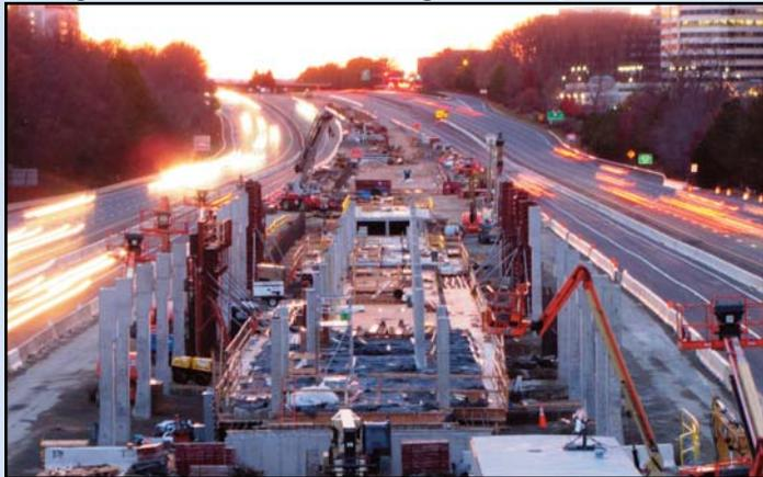
WIEHLE AVENUE STATION RISING: Looking west in the foreground are the platform deck sections now in place as work continues at this station under construction in the median of the Dulles International Airport Access Highway just west of the Wiehle Avenue overpass. Photo by Chuck Samuelson, Dulles Corridor Metrorail Project
