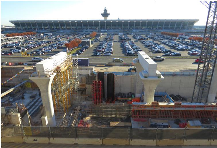
*The crossbeams pictured above will support Metro's Dulles Airport Station when complete and connect with the terminal, pictured in the background, via a pedestrian tunnel with moving sidewalks. (Photo by John Kearney, Dulles Corridor Metrorail Project)*
