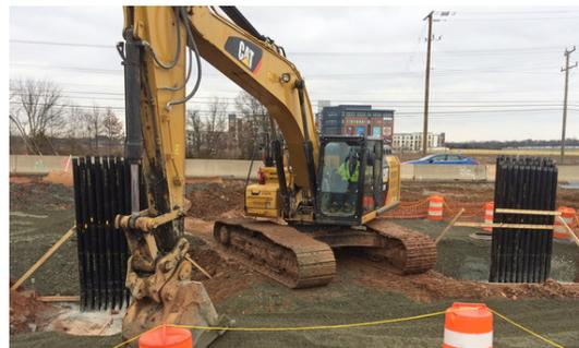
Electrical duct bank stub at the site of Ashburn Station in the median of the Dulles Greenway will contain and protect the power lines that will provide electricity to the station. (Photo by Richard Lynch, Capital Rail Constructors)
