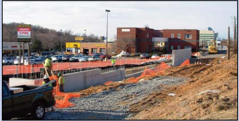
Construction of retaining walls on Route 7, necessary to build up the service roads to the same grade as Route 7 for lane shifting. Photo by Dulles Corridor Metrorail Project
