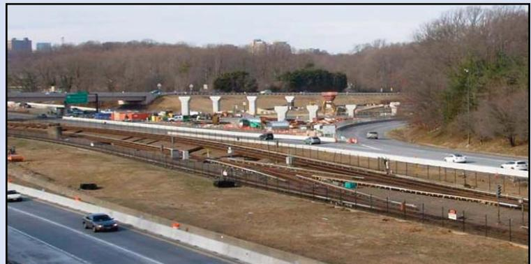
Pier guideway construction underway at the I-66 and Dulles Connector Road (Route 267) interchange. Photo by Dulles Corridor Metrorail Project
