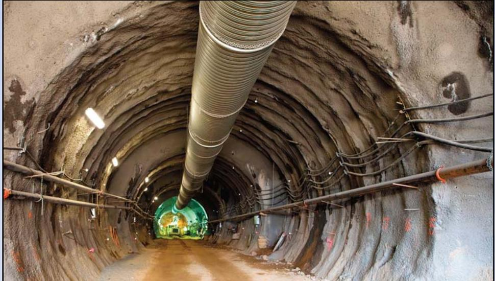
The outbound tunnel that will carry rail between Route 123 and Route 7 in Tysons Corner is currently 420-feet long and passes completely under International Drive. Photo by Rich Silva, Dulles Corridor Metrorail Project
