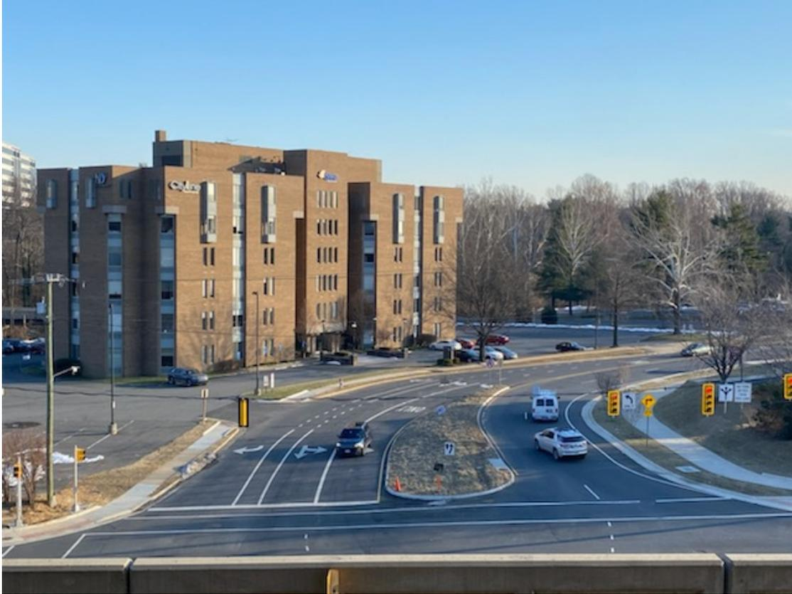
The realignment of Old Meadow Road, which was required by the state following construction of Phase 1 of the Silver Line, is now complete. While the final paving was done in November 2020, several minor punch-list items were required to finalize the work.
